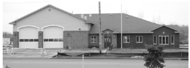
Manitowoc Road Fire Station
